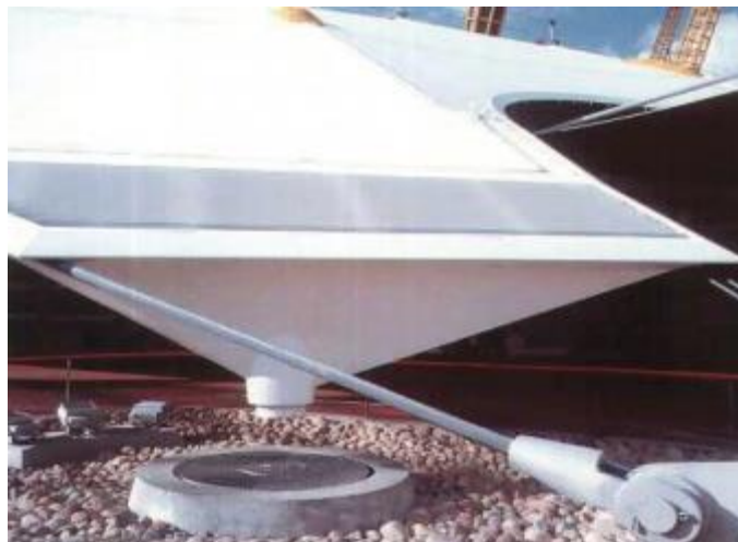
View of the entry to the rainwater storage system
